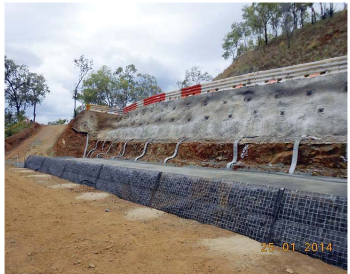
Above: works conducted at the Mount Morgan Range - reinforced earth embankment. Photo supplied.
