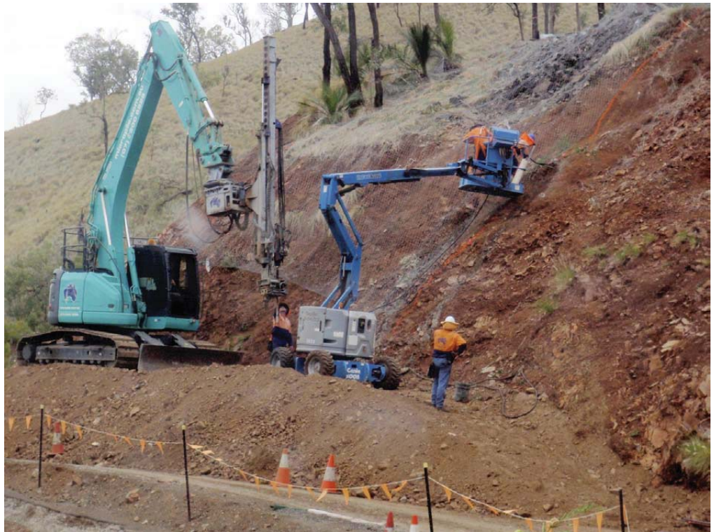
Above: works being conducted at the Mount Morgan Range - soil nailing and netting. Photo supplied.
