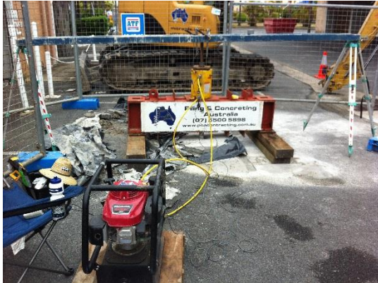
Load testing micropiles prior to final design
