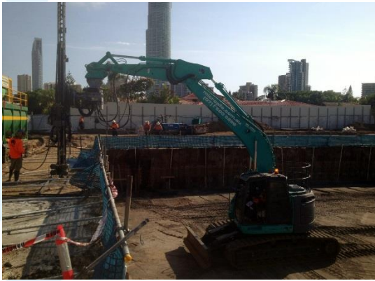
Installing micropiles from lower basement level into upper basement level
