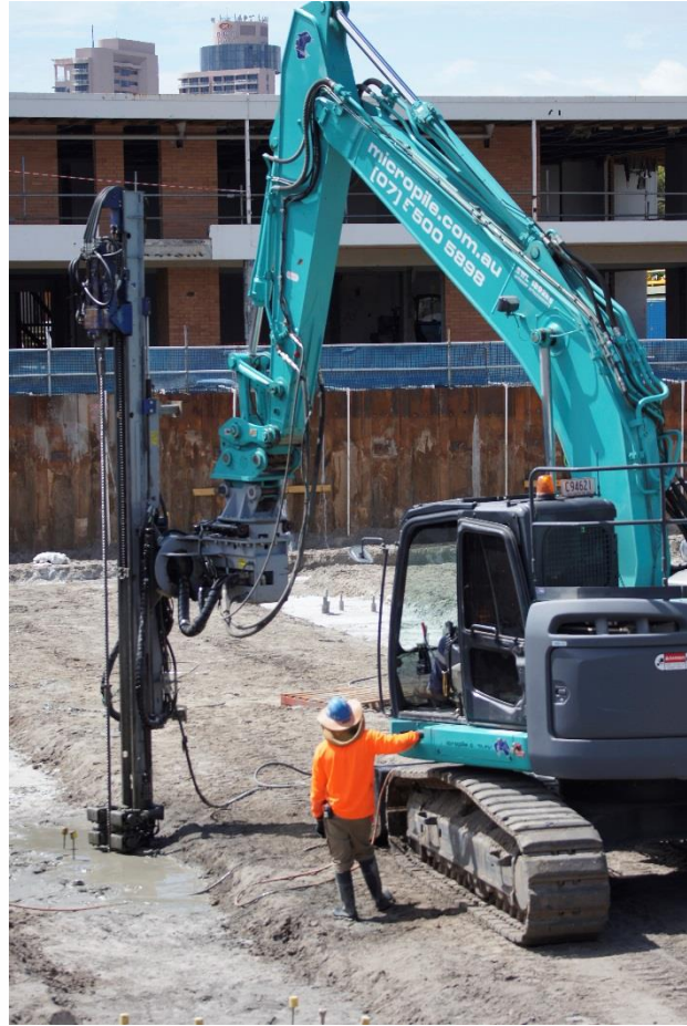
Installing micropiles in lower basement
