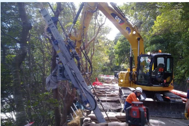
Precision angles on raked piles
