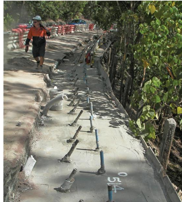
One lane of traffic remained open during construction
