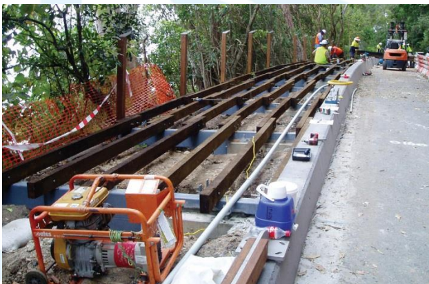
New boardwalk under construction
