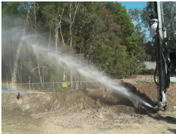
High pressure grouting was used to increase micropile diameters in upper soil layers
