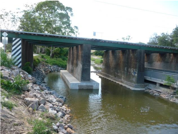
Completed foundation repair
