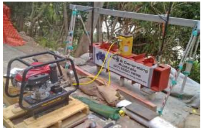
Piles were load tested to confirm design assumptions
