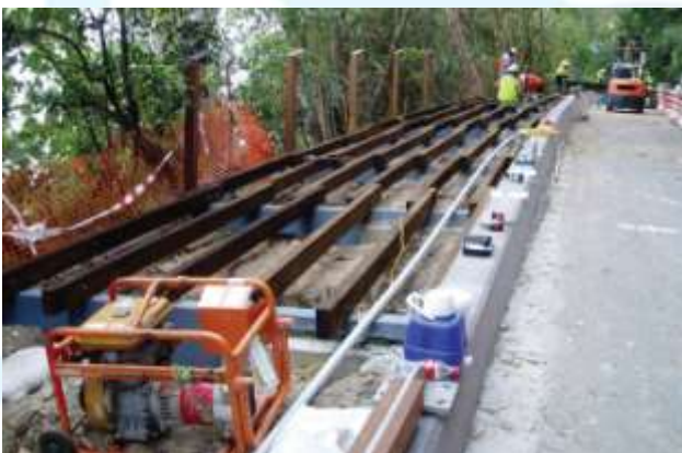
New boardwalk under construction
