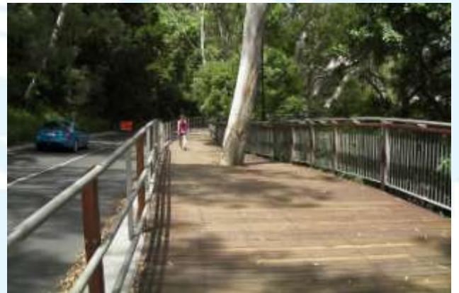
Noosa Boardwalk Completed
