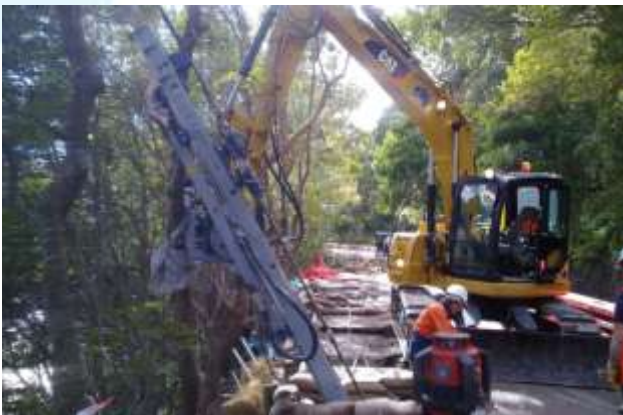
Precision angles on raked piles
