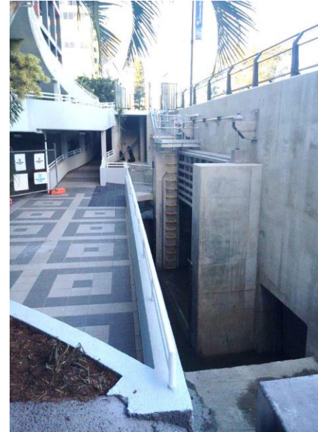
Completed works on right demonstrating the tight access conditions of the project
