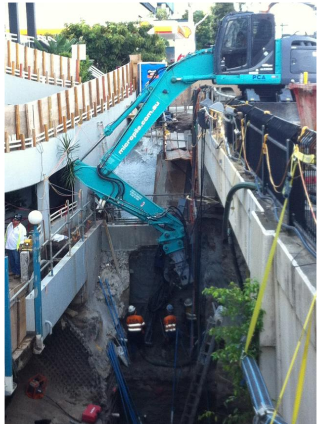
PCA's excavator mounted drill rig reaching down to install micropiles from the pedestrian lane adjacent Coronation Drive
