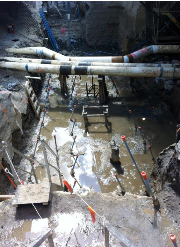
Micropiles installed in the foundation at opposing rake angles to handle the compression, tension and lateral forces
