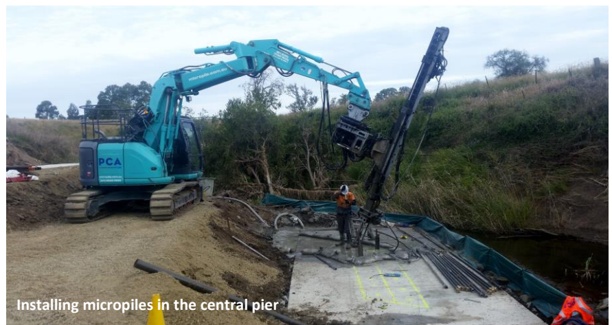
Micropiles installed in the central pier pile cap with column extensions for mid span headstock
