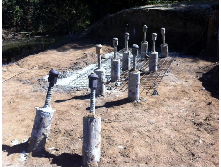
Raked and vertical micropiles installed in abutment location
