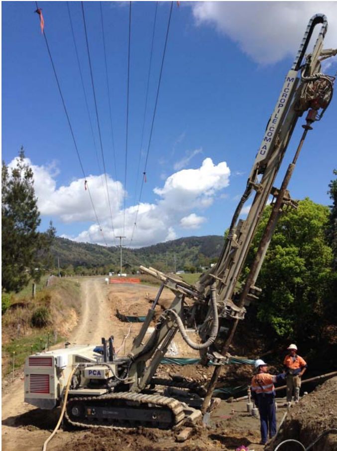
Installing raked micropiles in close proximity to powerlines
