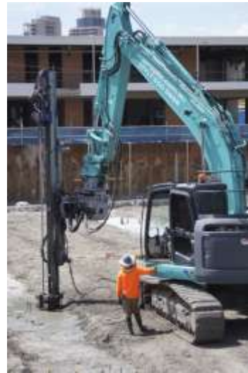
Installing micropiles in lower basement
