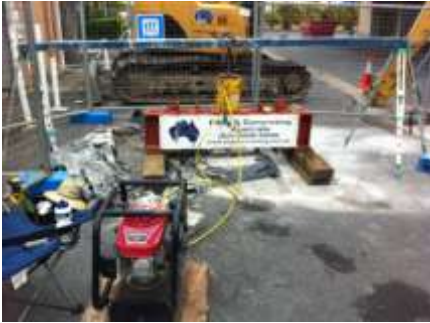
Load testing micropiles prior to final design
