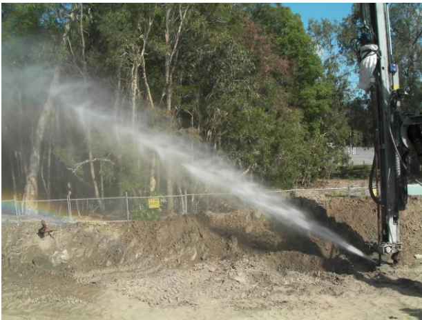
High pressure grouting was used to increase pile diameters to 400mm.
