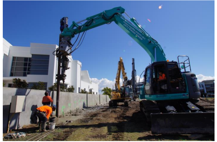
Installing the 6m long universal beam
